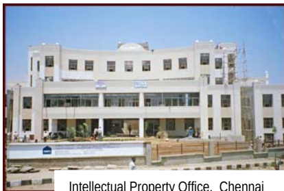
Intellectual Property Office, Chennai
